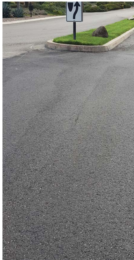
After: Road repaired
