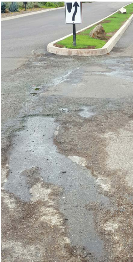
Before: Road damaged by water runoff
