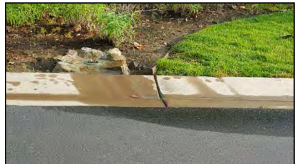
Excess watering visible at drain outlet
